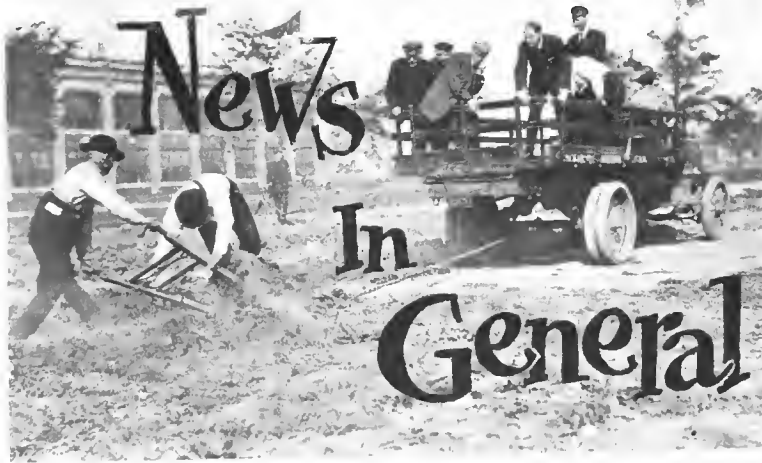
How the Packard Truck Was Utilized to Break Ground for Factory Addition.
